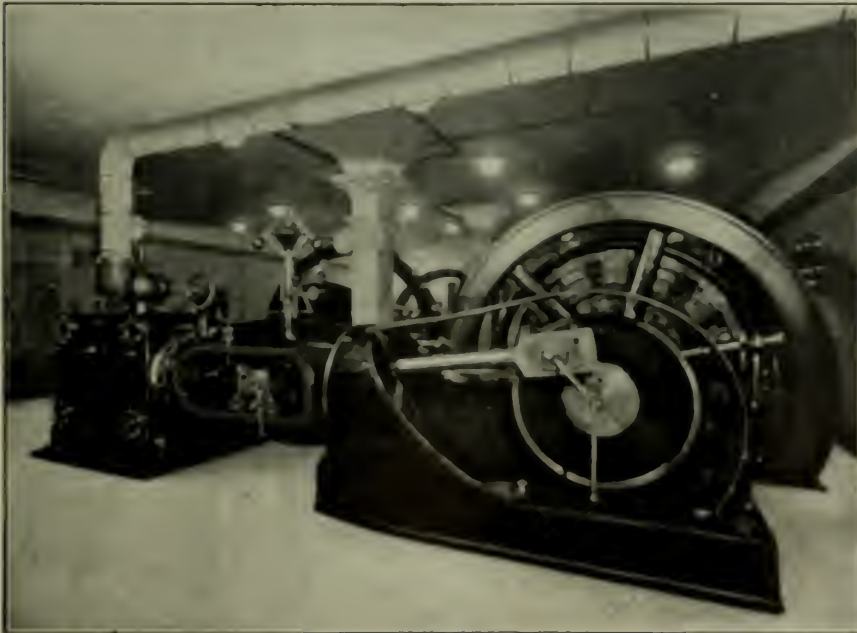
FIG. 4. ANOTHER VIEW OF THE ENGINE ROOM
